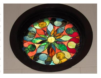
The window is 38 ½ inches in diameter. The original carpenter building the church had the forethought to install the window so that it could be removed without destroying the circular molding that held it in place. The workers were surprised that it was such a straight-forward process.
