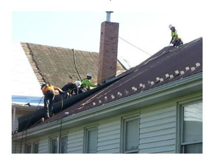
Here, you can see the workers from Kruger Roofing, as they remove a sheet of old metal roofing. You can see sections of the original skip sheeting on the roof over the gym, with the first 2 layers of old roofing (cedar shakes, then a composition shingle). You also see the new water and ice shield that has been applied over the new plywood decking on the left, awaiting the new and heavier, 26
