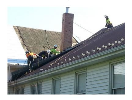
Here, you can see the workers from Kruger Roofing, as they remove a sheet of old metal roofing. You can see sections of the original skip sheeting on the roof over the gym, with the first 2 layers of old roofing (cedar shakes, then a composition shingle). You also see the new water and ice shield that has been applied over the new plywood decking on the left, awaiting the new and heavier, 26
